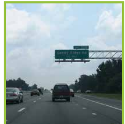
Sandy Ridge Road serves as the main southern gateway from I-40 into the Western Area.
