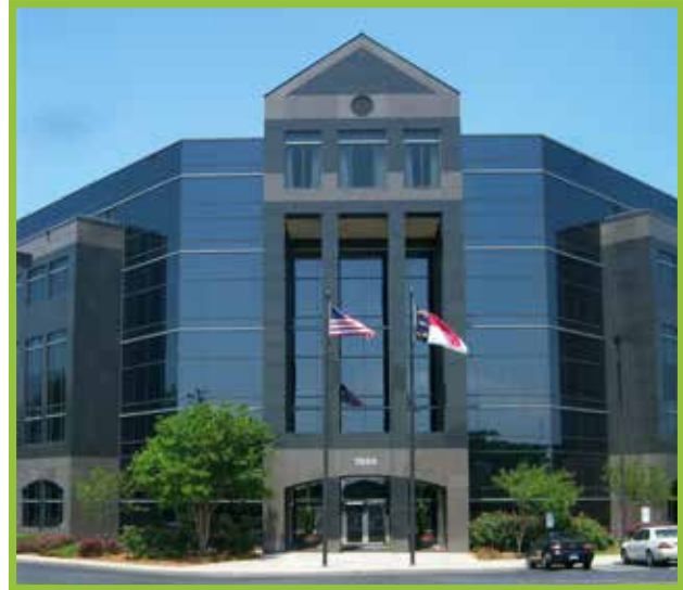
As a strategic location in North Carolina for employment, office square footage in the Western Area will double by 2030.
