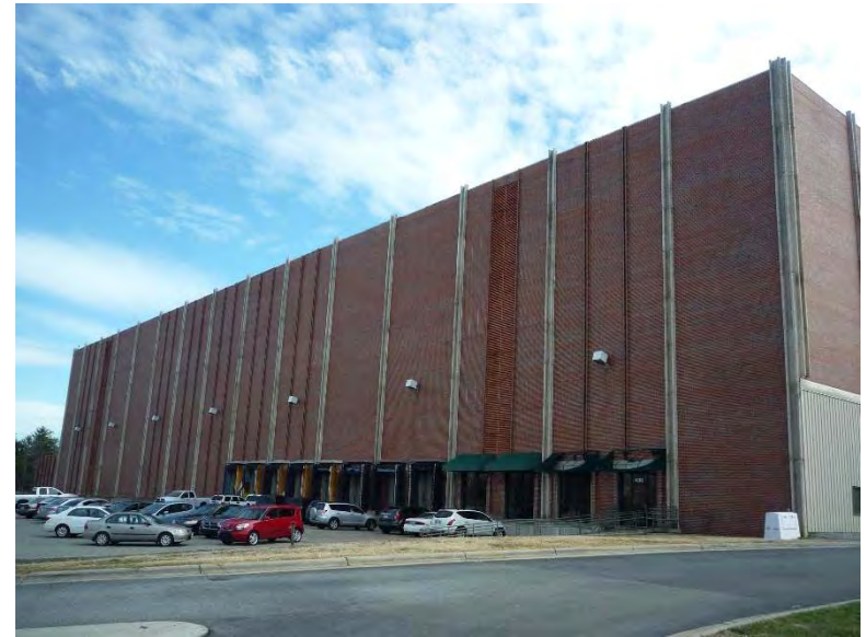
Loading docks of Sears Building, currently in use by Loomcraft Textiles.
