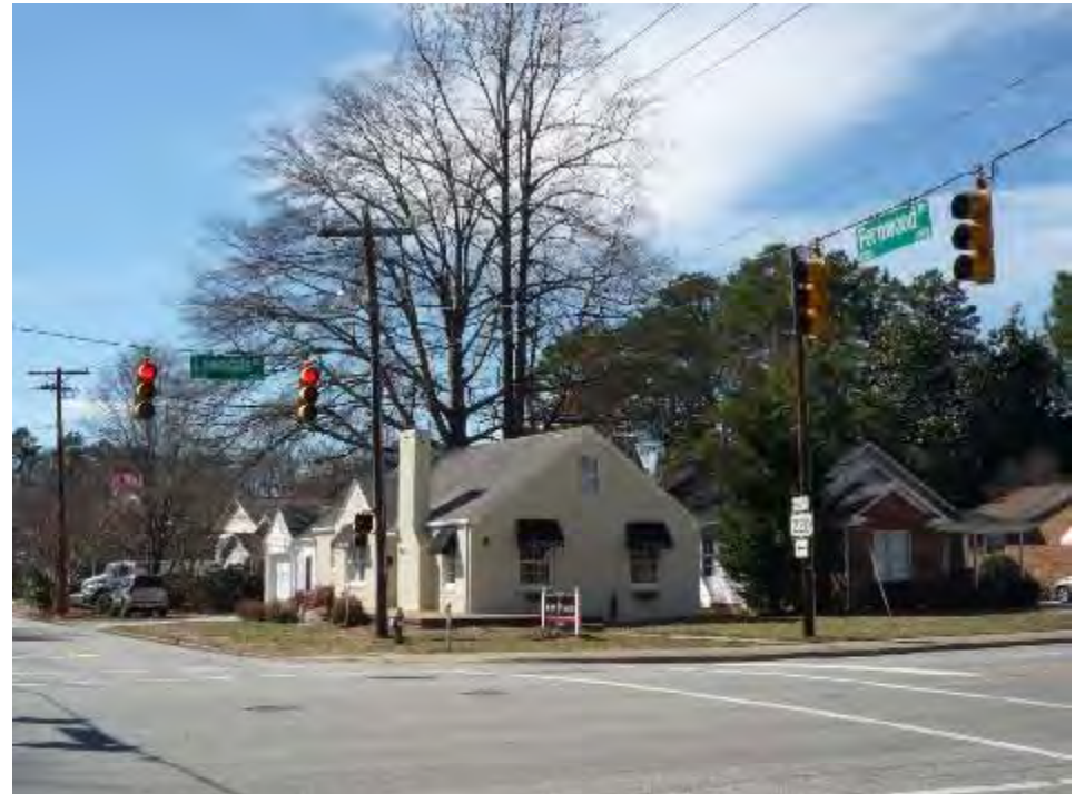
Recent commercial adaptive reuse at the corner of Lawndale Drive and Fernwood Drive.
