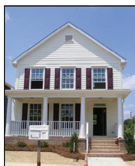
Phase II Construction
