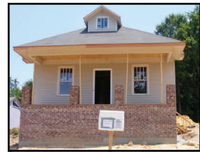
New Single Family Home Construction by Self-Help
