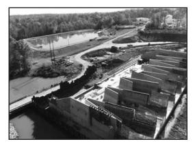
Townsend Dam, Greensboro's major water supplier, is getting a much needed facelift. The 1,635-acre water source has supplied 70 percent of the City's water since the 1960s. The dam is also used for recreational boating and fishing. Signs of structural distress became evident in 1980 due to Alkali-Silicia Reactivity (ASR), which made renovations a necessity. If left
