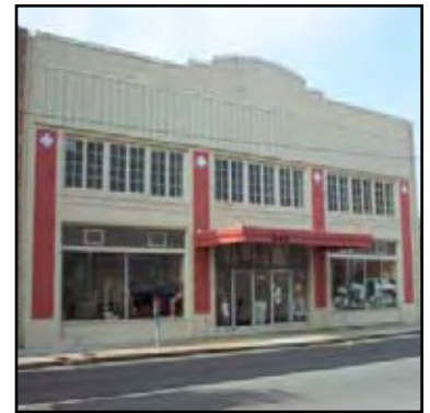
The entrance to this building uses a canopy structure and an accented parapet to give an unassuming entrance more prominence.
