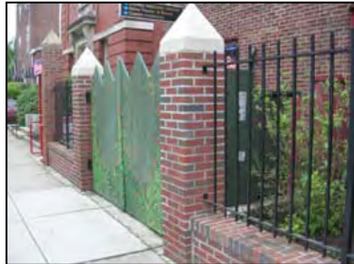
While this waste receptacle is located directly adjacent to the sidewalk, the decorative screening mitigates the receptacles unsightly elements.
