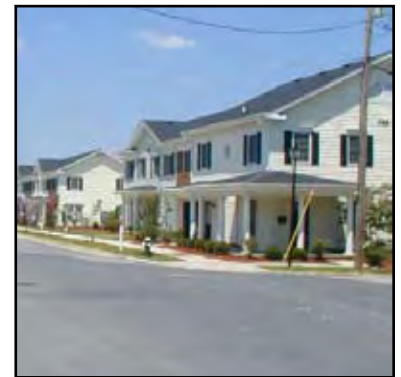
These joined town homes have their long elevations oriented toward the street, providing a greater presence and visual interest to pedestrians.
