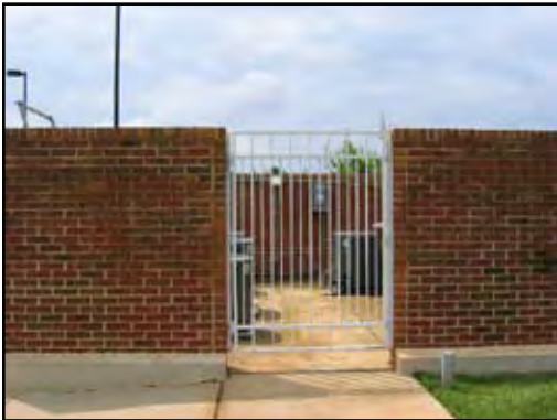
The brick screening and decorative wrought iron gate screens building utilities in a parking lot.
