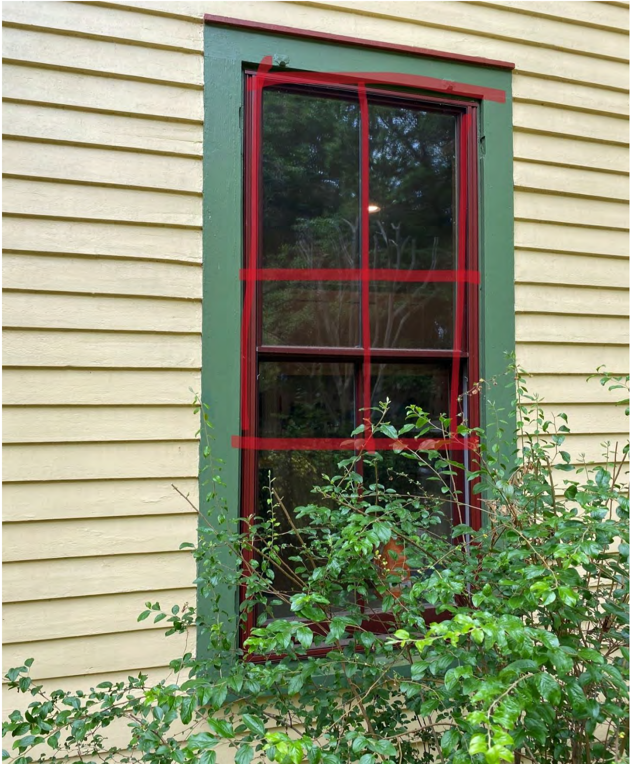
Figure 37 – 924 Carr St shorter window installed on rear elevation to accommodate sink
