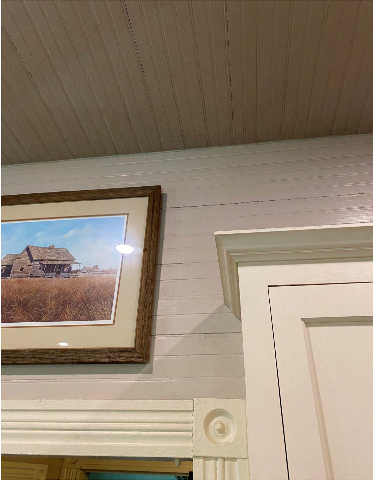
Figure 29 – 924 Carr St bead board and mouldings to be reused
