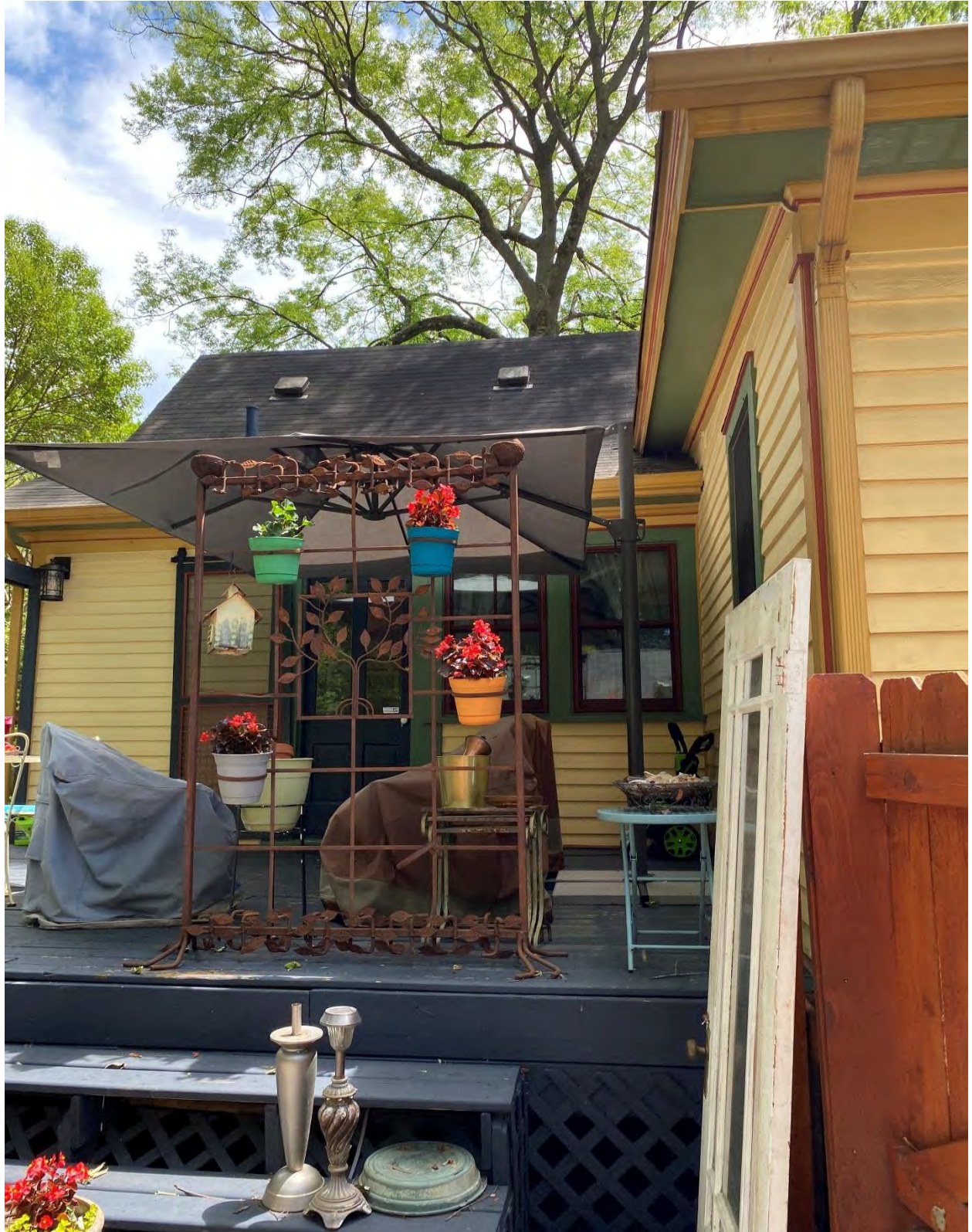
Figure 21 – 924 Carr St. rear side entrance not visible from street
