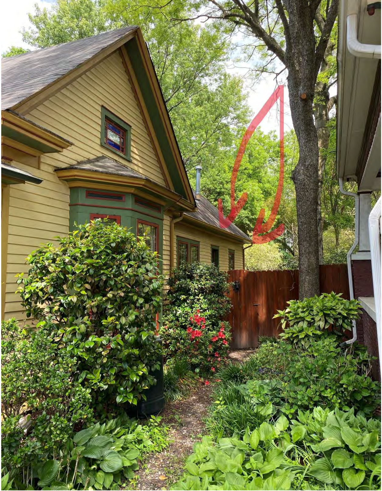
Figure 42 – 924 Carr St replacement windows from near street, obscured by fence
