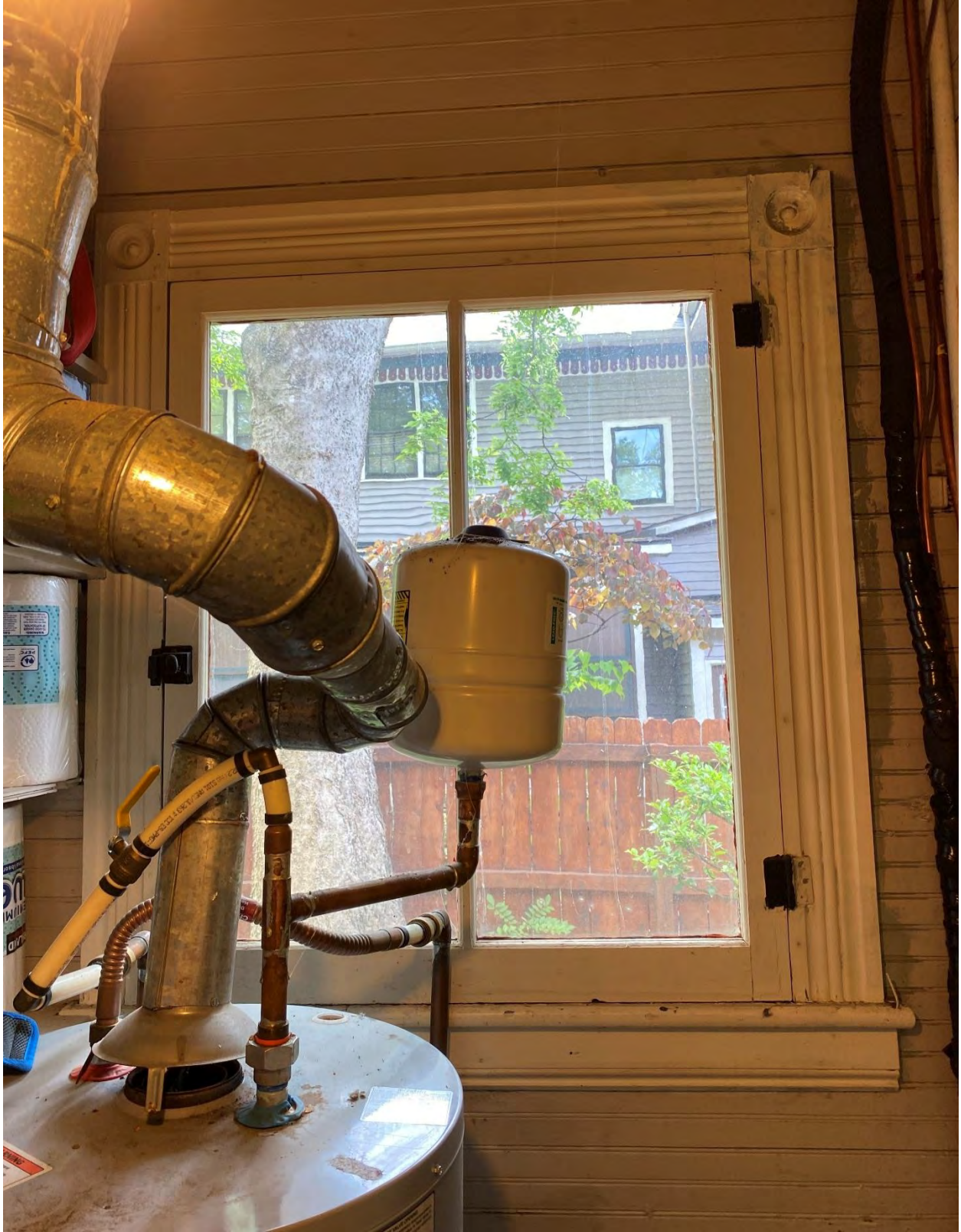
Figure 18 – 924 Carr St. broken window in unheated storage room
