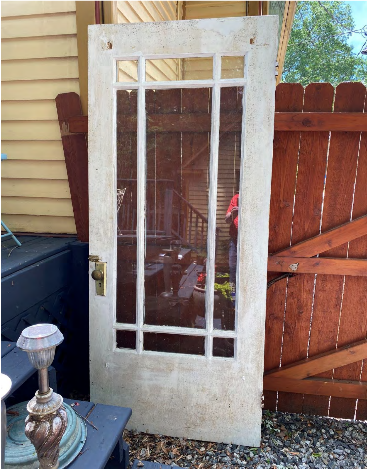
Figure 44 – 924 Carr salvaged period door to replace inappropriate rear side entrance door
