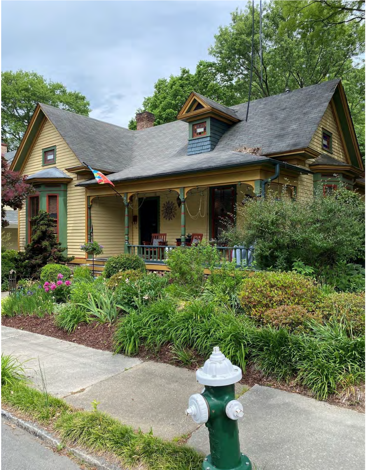
Figure 1 – 924 Carr St. carefully preserved
