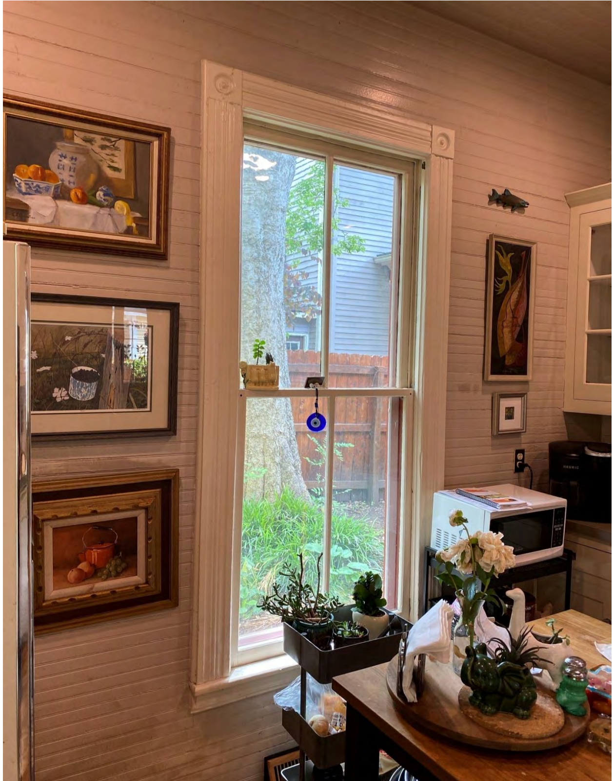
Figure 11 – 924 Carr St. side elevation reworked window, possibly not original location
