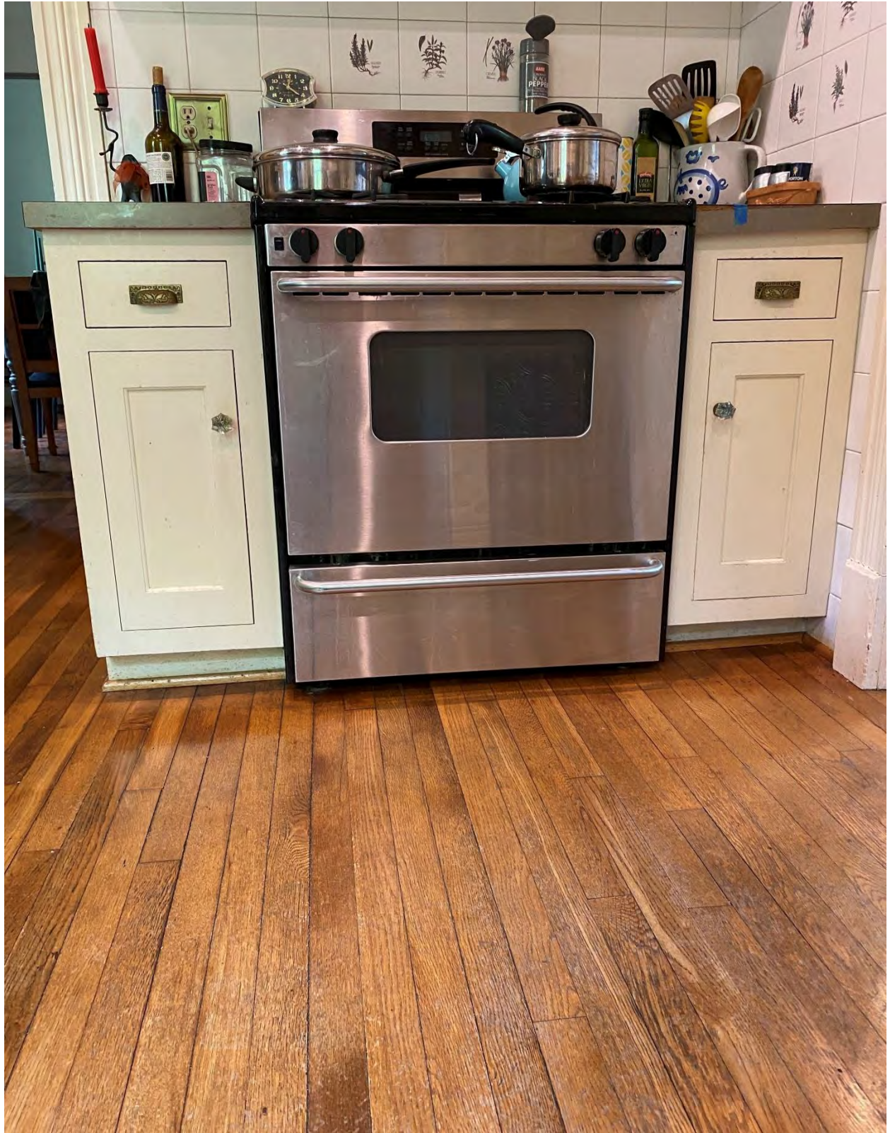
Figure 32 – 924 Carr St site-built cabinets to be relocated
