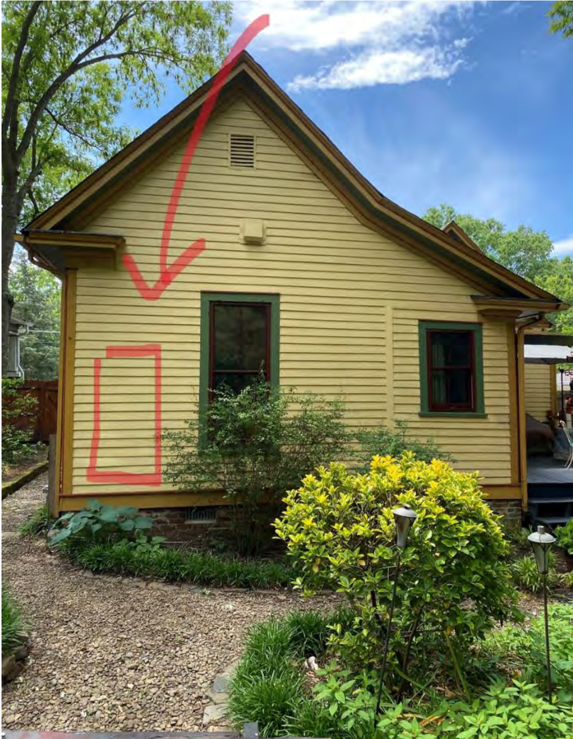
Figure 34 – 924 Carr St tankless water heater installed on rear elevation
