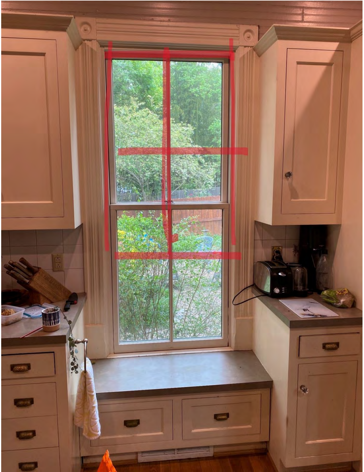
Figure 36 – 924 Carr St shorter window installed on rear elevation to accommodate sink
