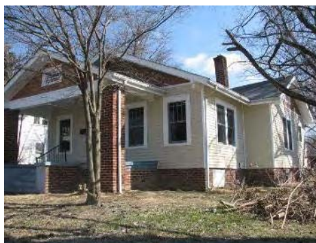
1603 Randolph Avenue after rehabilitation
