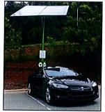
**T1** - Our 2 kilowatt Brightfield® provides 10,000 miles of solar fuel annually and can accommodate up to 3 Level-2 chargers. This system is ideal for lower frequency or congested sites.
