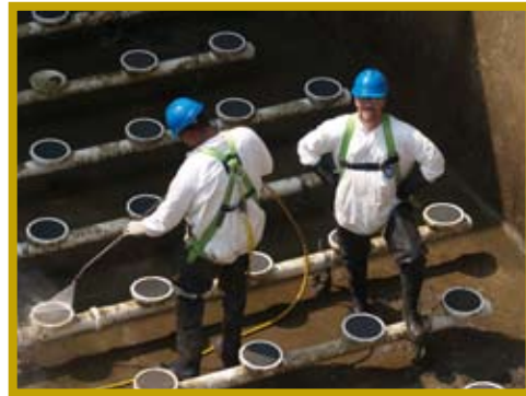
Routine facility maintenance by wastewater staff
