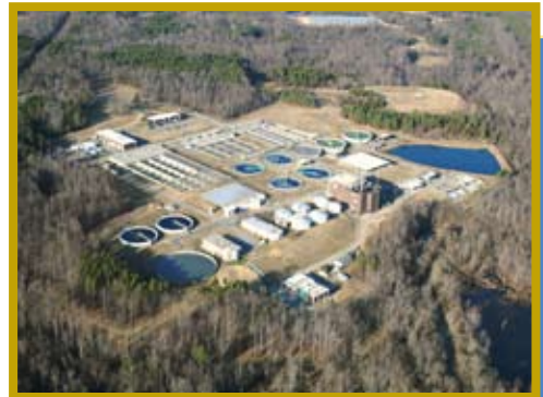
Aerial photo of T. Z. Osborne Plant (located off of Huffine Mill Road)
